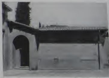
Fig. 106. S. Sebastianus' Perimeter, part of basilica opus testatum and under south wall of Mausoleum of the First Sacristy.
